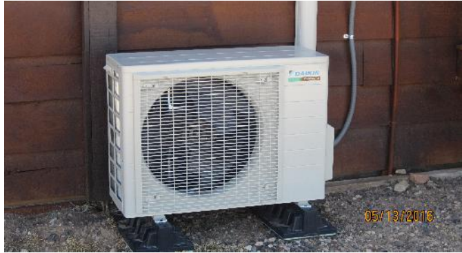
The air conditioner outside the building was replaced in 2015.
